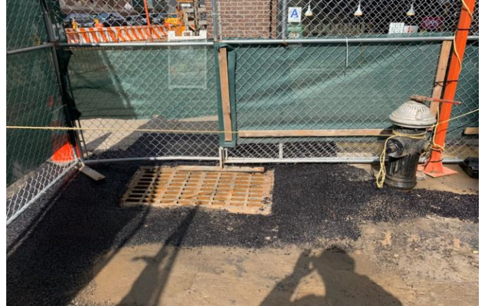
Newly installed catch basin on E. 25 th Street and Lexington Avenue
